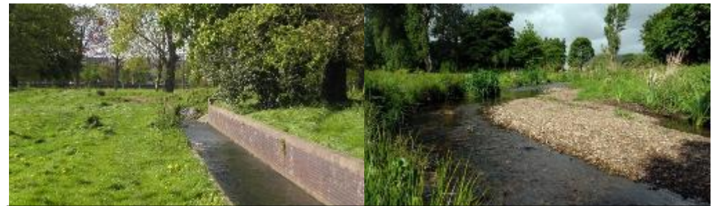
Inch Park – moving away from hard flood prevention measures to more naturalised solutions
